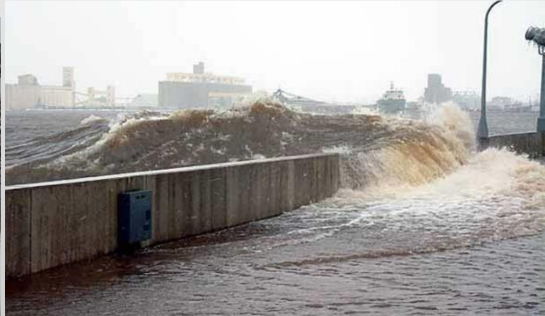
Wind-generated waves breach the harbor structure in Canal Park in Duluth, Minnesota. (Source: Gene Clark, Wisconsin Sea Grant)
