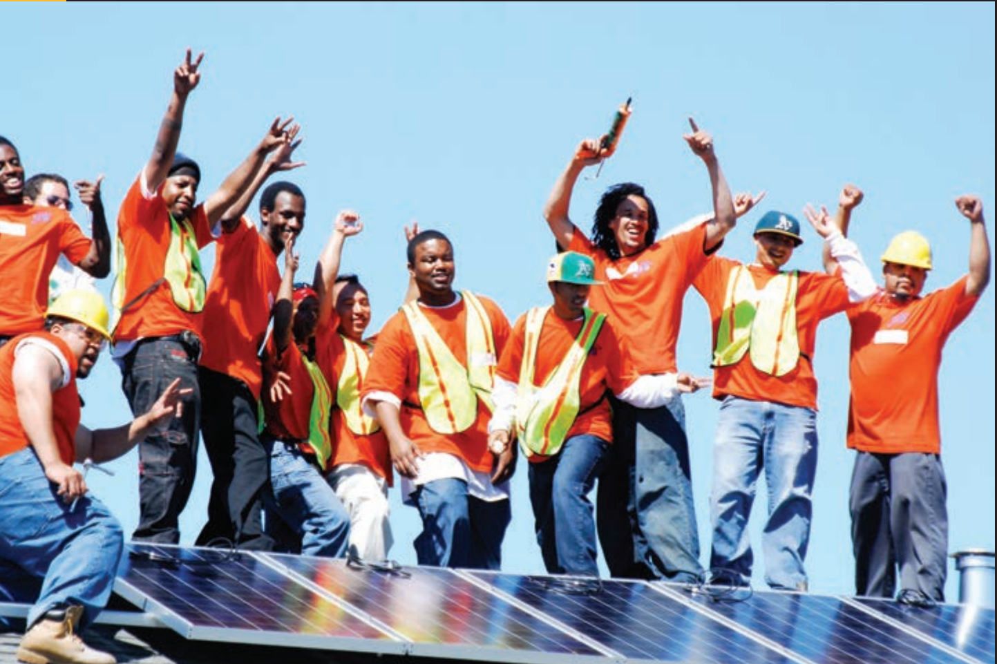
Job trainees get hands-on experience installing a solar electric system for a low-income homeowner in Richmond, CA. Photo: Solar Richmond and Green for All.
